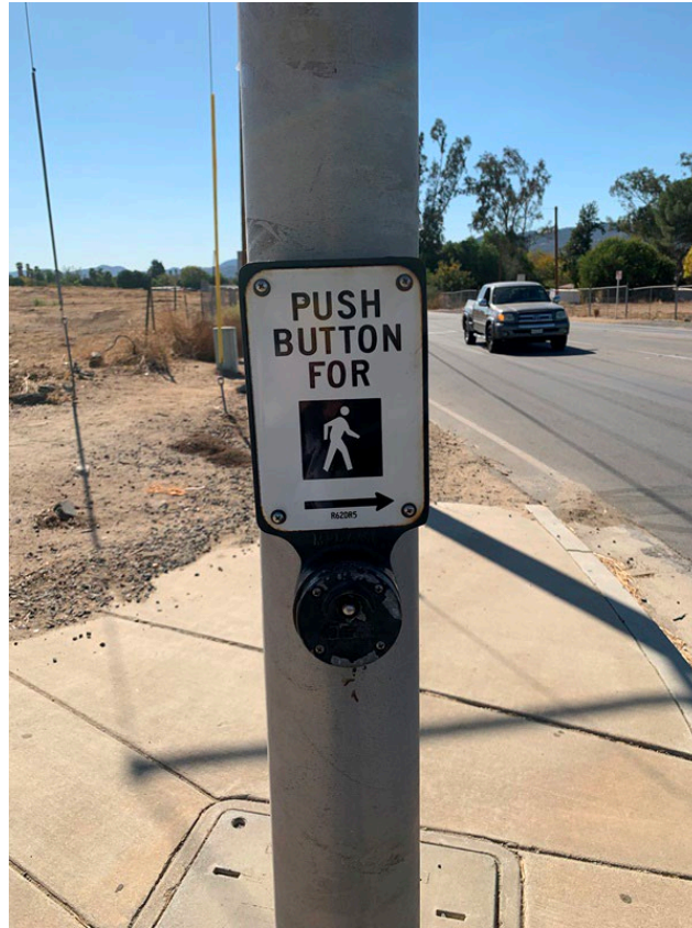
Figure 3.5: Non ADA-Compliant Pedestrian Push Buttons
