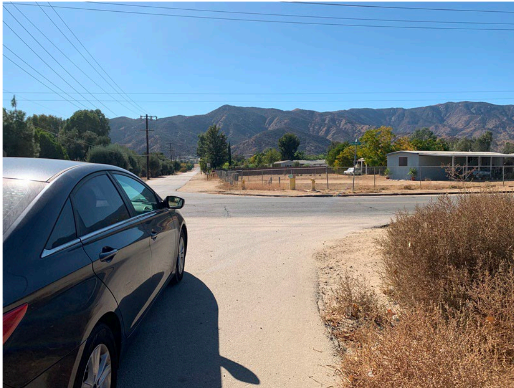
Figure 3.14: Missing Stop Sign and Pavement Markings on the Bryant Street North of Palomar Street
